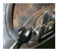
Next, align the screw hole on the inlet side of the float holder and the bottom hole of the plate, and temporarily tighten the hexagon bolt with a spanner, ring wrench, etc (width across flat: 13 mm). The plate will be on the upper side of the float holder as shown in the picture.
